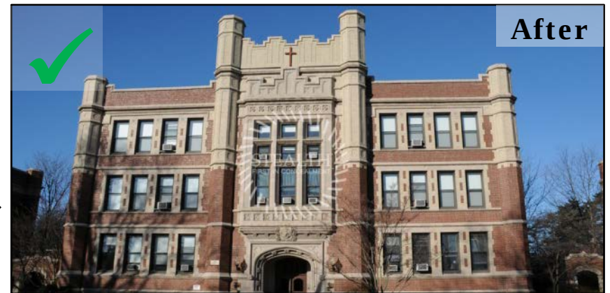
Figure 8 – Building after construction of extended parapet serving to conceal a new roof-mounted facility.
