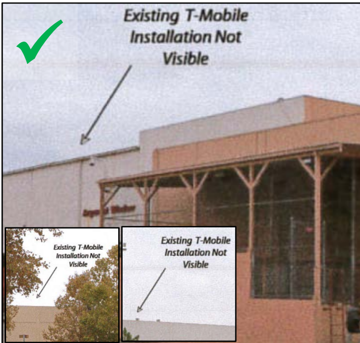
Figure 4 – Example of a facility which is imperceptible to the public from multiple vantage points, as a result careful placement when considering the height of the equipment.
