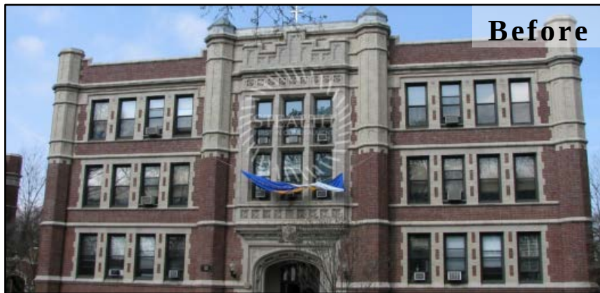
Figure 7 – Building prior to construction of concealment.
