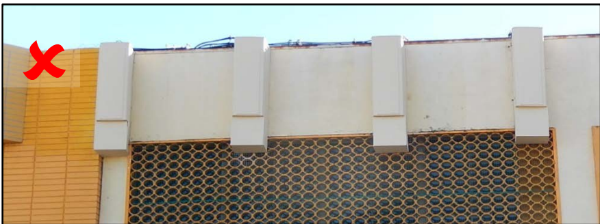
Figure 12 – Unsuccessful example of antennas trying to replicate an architectural feature. These antennas extend above the parapet of the building, and protrude down in front of a metal mesh screen.
