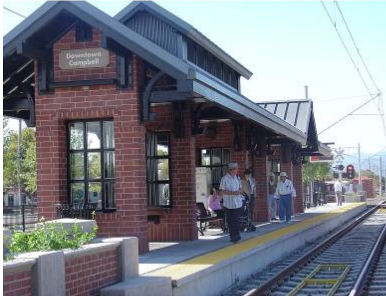
Downtown Campbell Light Rail Station
