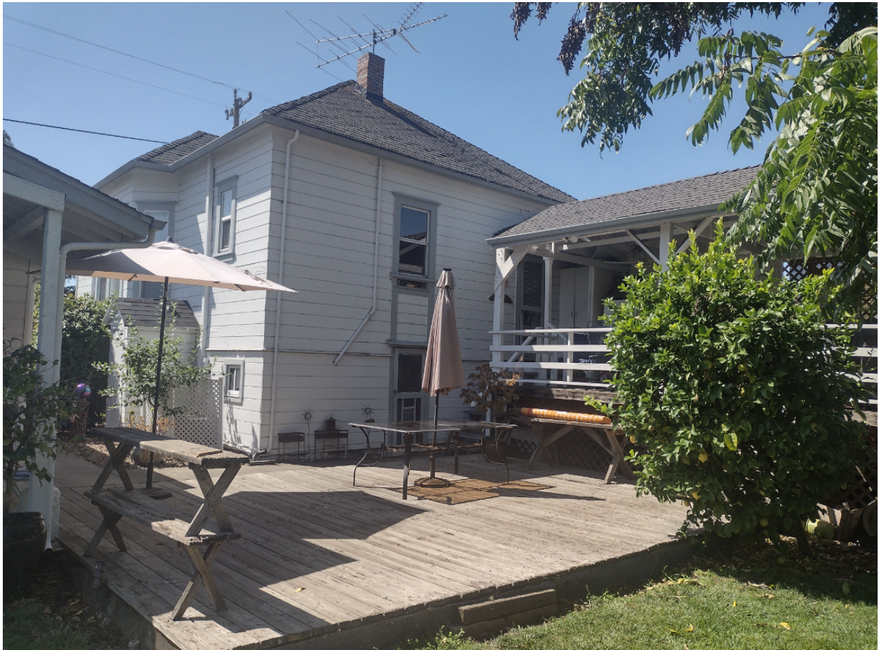
Figure 7. North facade, view southwest
