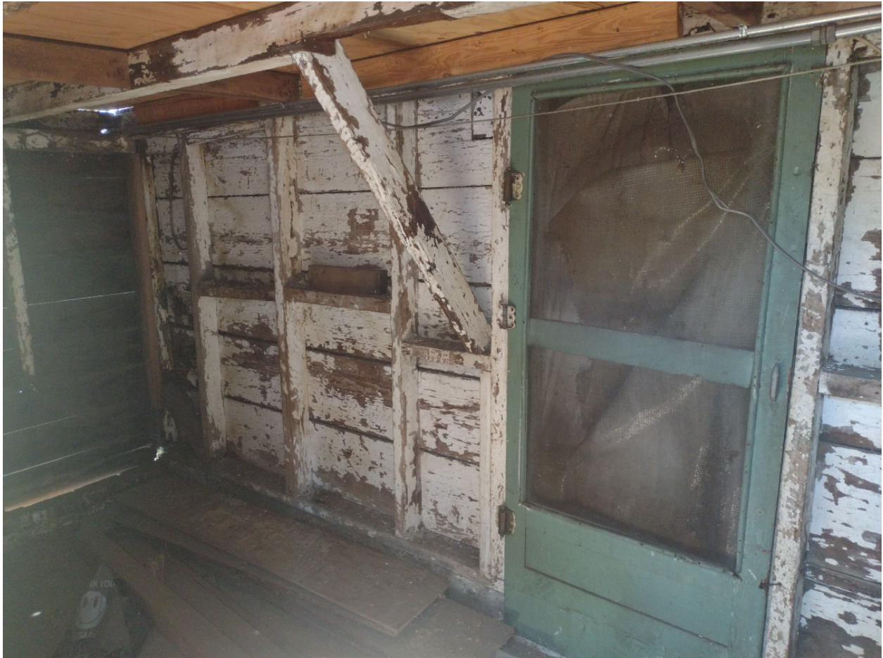
Figure 15. Underneath the porch
