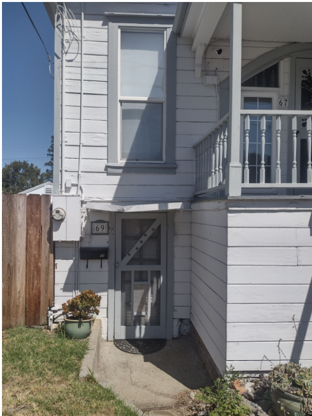
Figure 5. Close-up of South Facade, facing north
