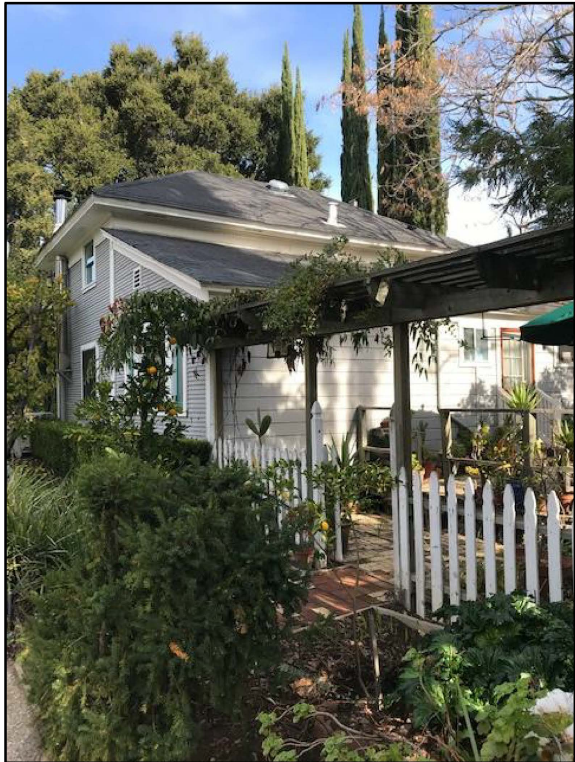
PHOTOGRAPH 5: VIEW LOOKING AT THE PROJECT'S WEST AND SOUTH EXTERIOR ELEVATIONS
