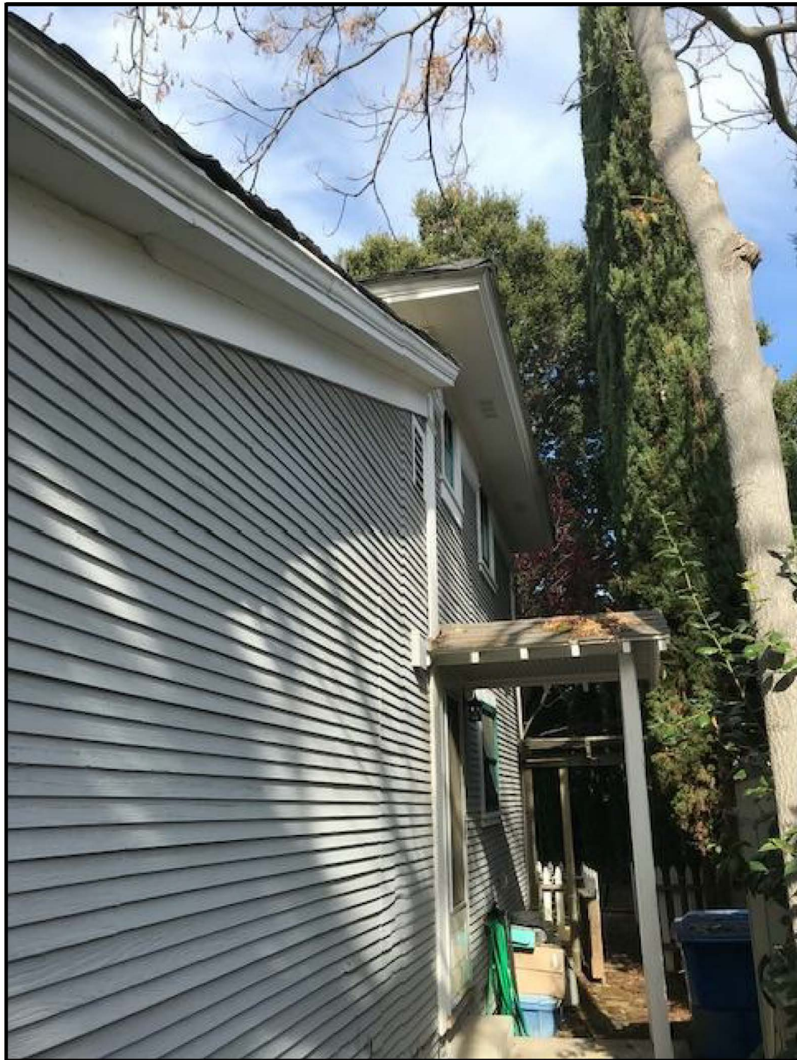
PHOTOGRAPH 4: VIEW OF THE EXISTING EAST EXTERIOR ELEVATION
